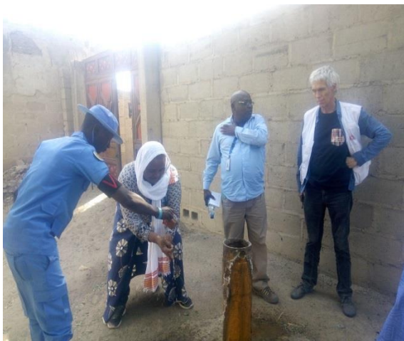
Inspection of borehole
